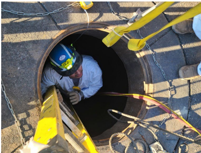
Figure 6.1 Tucson Water Staff at Work
