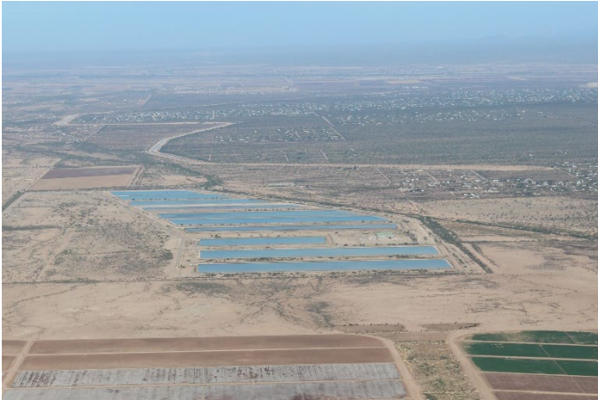
Caption: Aerial view of Tucson Water's Central Avra Valley Storage and Recovery Project facility
