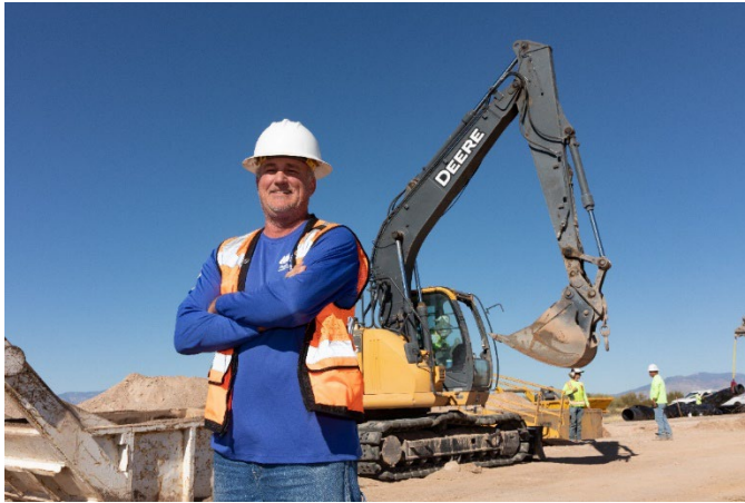
Figure 6.2 Tucson Water Staff at Work
