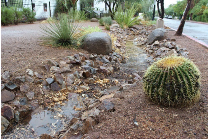
Caption: Green Stormwater Infrastructure, can reduce flooding on streets and often divert that water into basins to irrigate vegetation that can shade streets and sidewalks.
