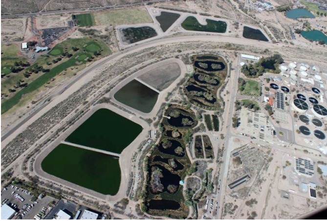
Caption: Aerial view of the Sweetwater Recharge Facility and Wetlands.
