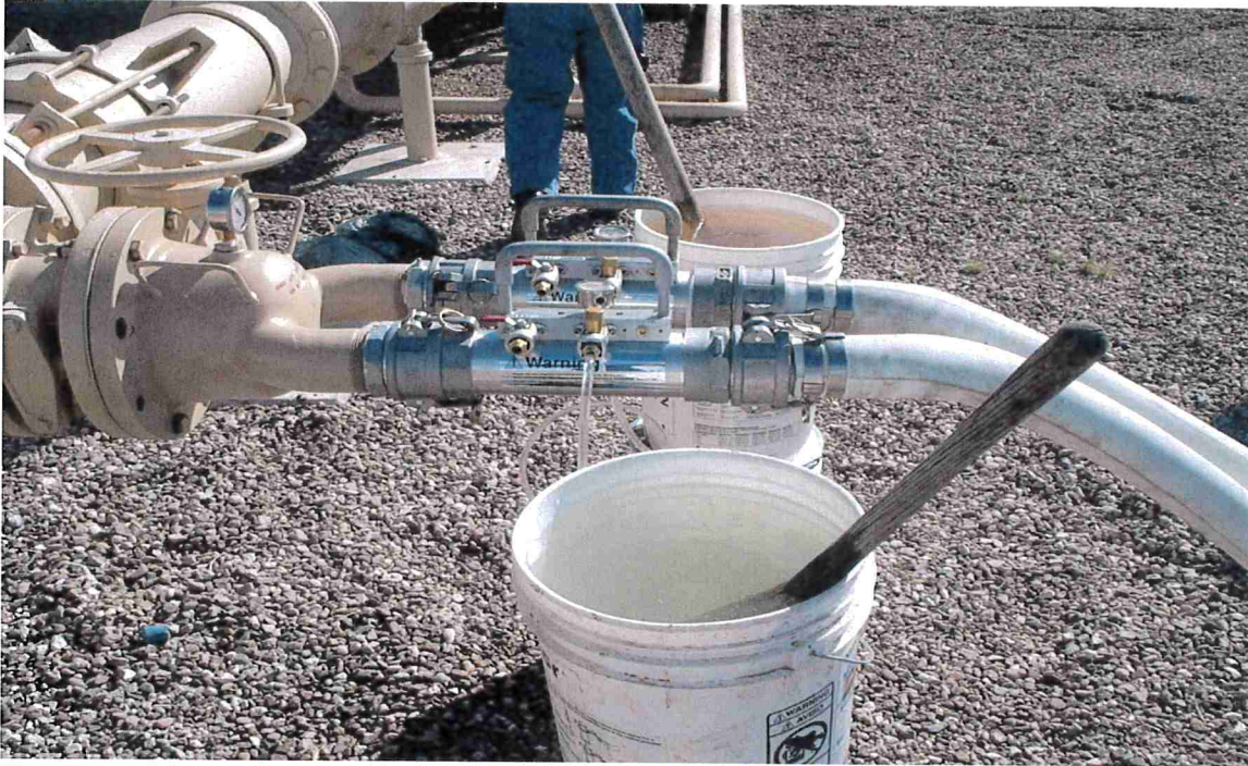
Two Venturi Manifold for flows greater than 1800 GPM – CA-009A De Chlorination Image from Andrew Vanover , Tucson Water.
