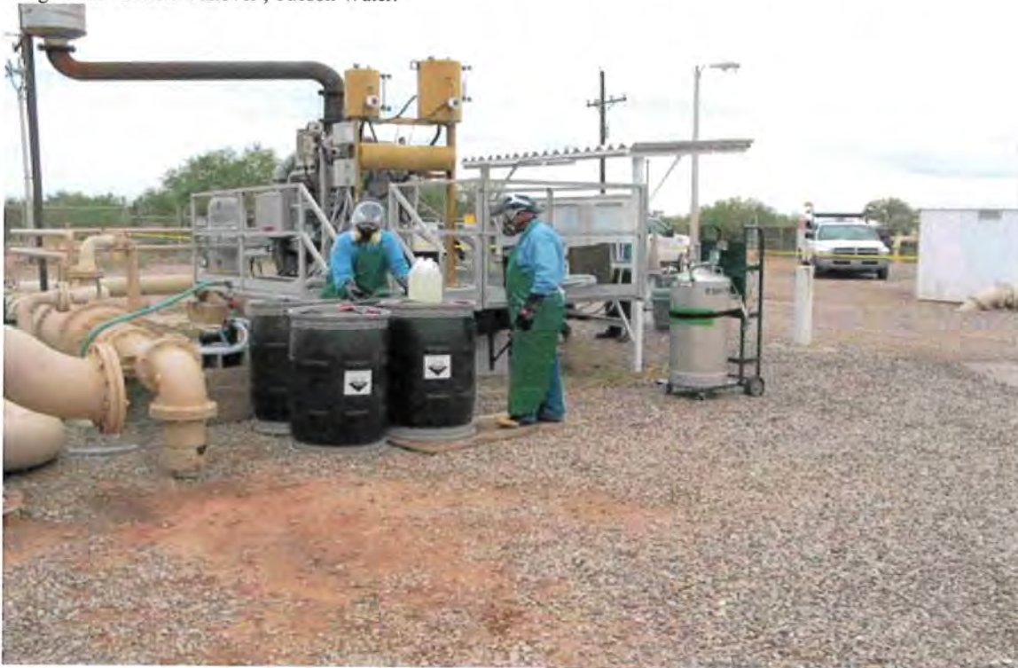
Sodium Bisulfite is used to de-chlorinate discharges over 200 ppm Image from Laura Macklin, Tucson Water.
