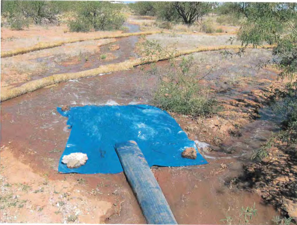
Straw Wattles and the discharge lay flat at the 36 inch main dewatering.
