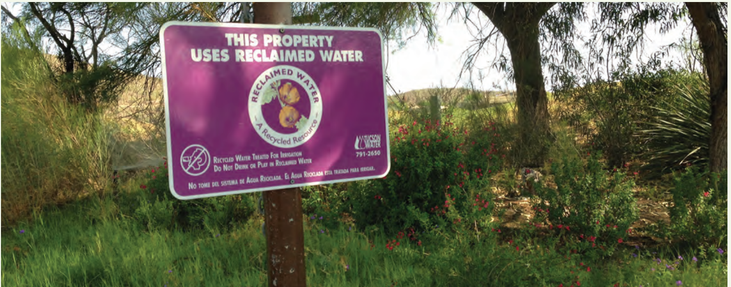
SIGNAGE FOR THE RECLAIMED WATER SYSTEM
