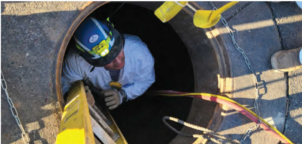
TUCSON WATER STAFF AT WORK
