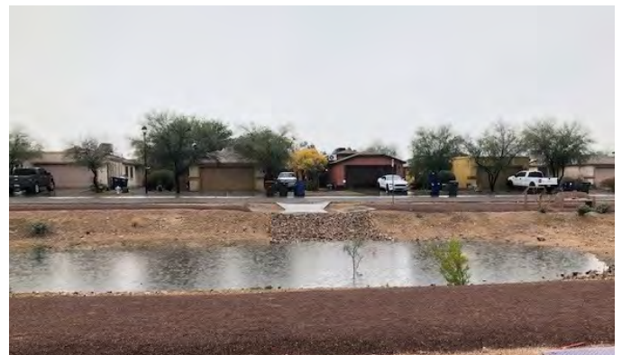
Stormwater capture in action at Sunland Vista Wash
