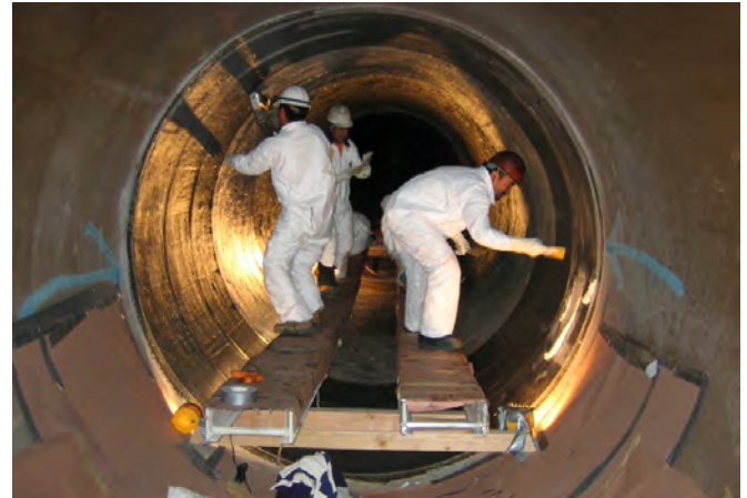
96" pipeline repair
