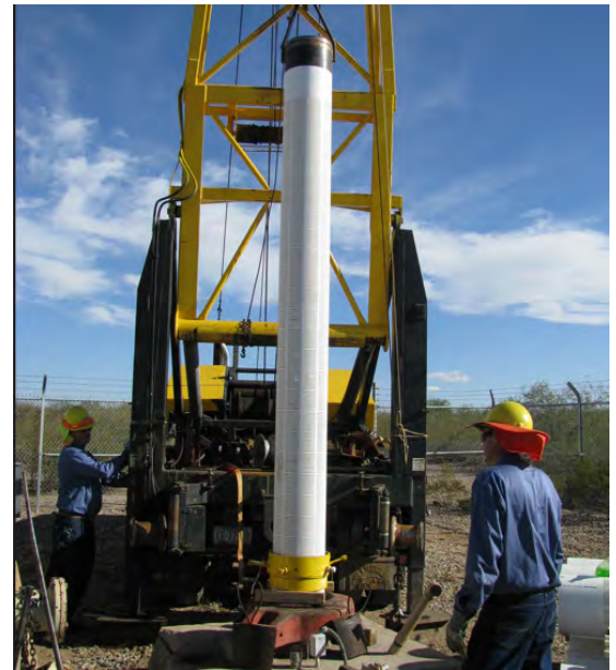
Tucson Water staff installing a new screen at well SC-003A
