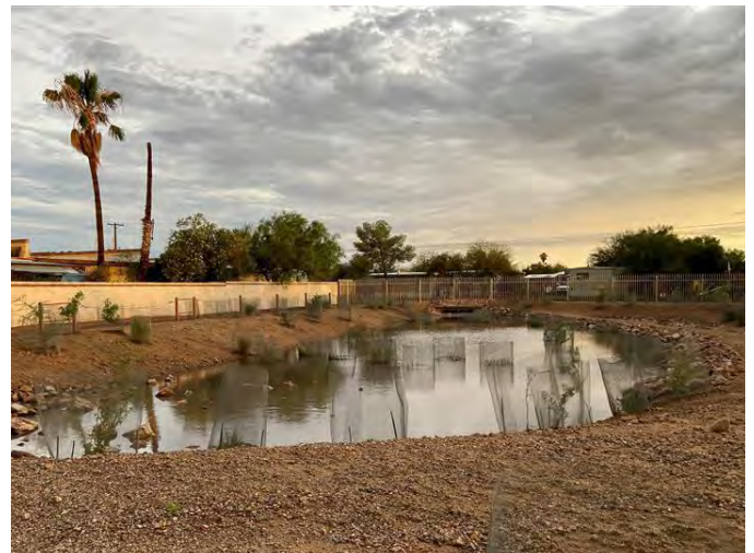
Cherry Avenue storm water capture project captures and retains up to 77,049 gallons of stormwater in a two-cell vegetated basin, mitigating nuisance flooding in the surrounding neighborhood.
