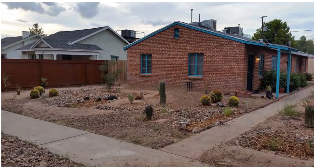
Residential rainwater harvesting
