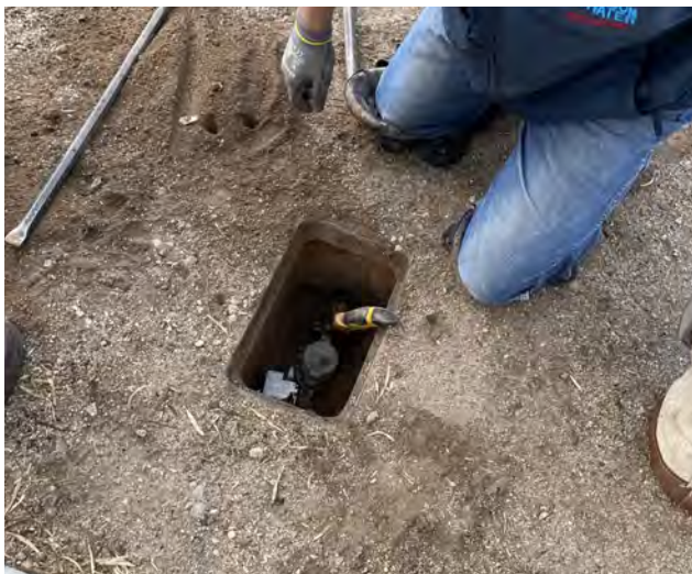
Tucson Water technician installing an ultrasonic smart meter
