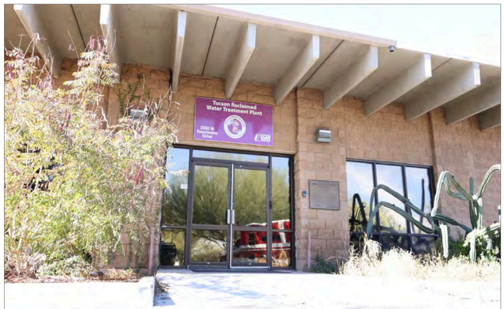
Tucson Reclaimed Water Treatment Plant
