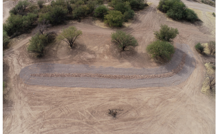
An aerial photograph of an infiltration trench installed in December 2024 to promote aquifer recharge at the Rita Ranch Detention Basin Project.
