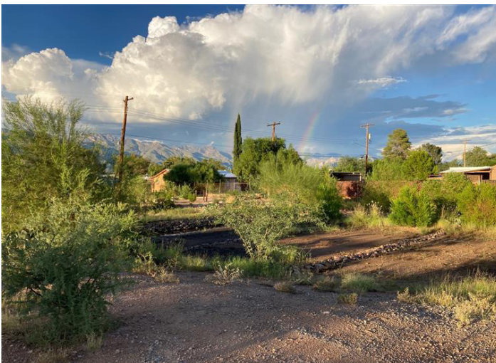
Seneca Basin was designed and constructed by Pima County on a 1.67-acre property to combat decades of flooding suffered by the surrounding neighborhood. The basin can harvest 321,662 gallons of stormwater flowing off Seneca Street. Seneca Basin was designated a City Park in 2022.
