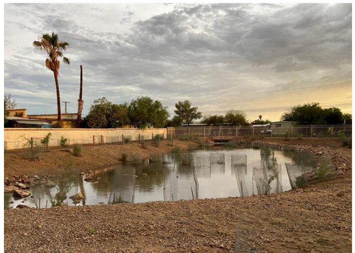
Cherry Avenue storm water capture project captures and retains up to 77,049 gallons of stormwater in a two-cell vegetated basin, mitigating nuisance flooding in the surrounding neighborhood.
