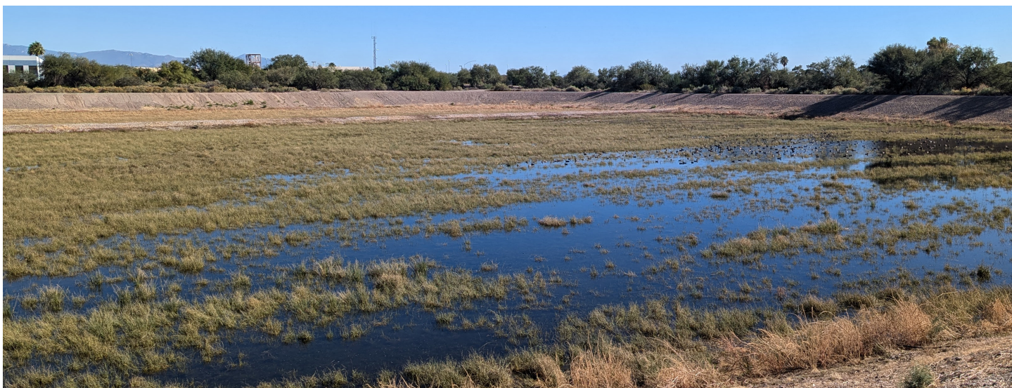
Recharge of reclaimed water at the Sweetwater Recharge Facility, Tucson's first recharge and recovery project.
