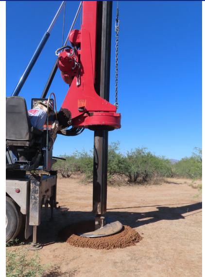
Tucson Water staff installing a new screen at well AV-001B
