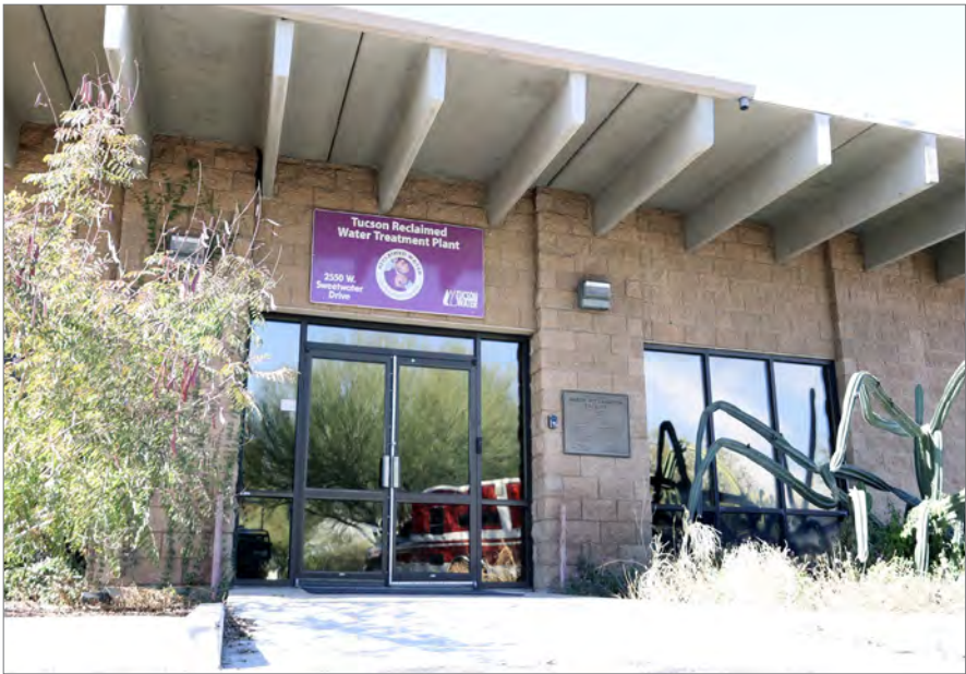
Tucson Reclaimed Water Treatment Plant
