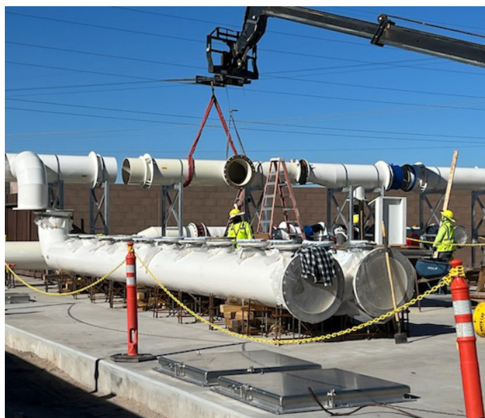
Installation of IX vessels at TARP
