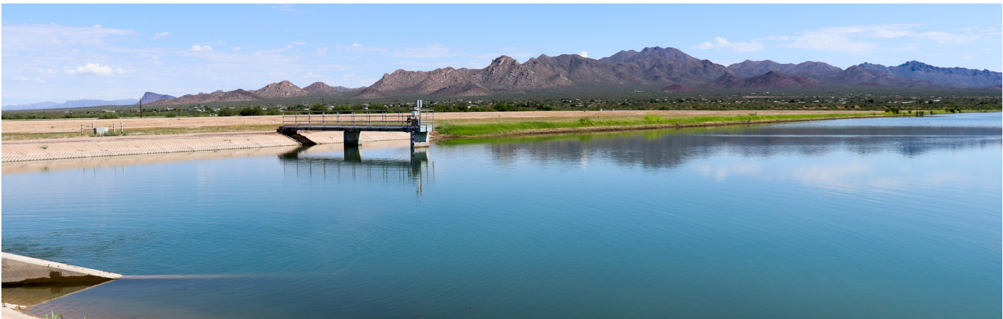
CAVSARP recharge basin, Water Bank of Tucson
