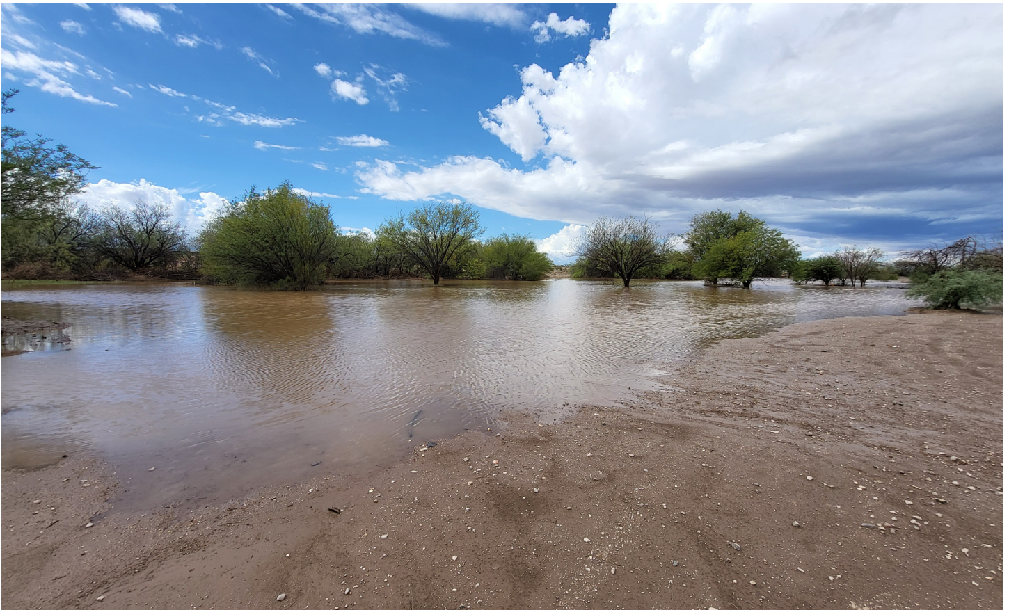
Rita Ranch Stormwater Site after precipitation event
