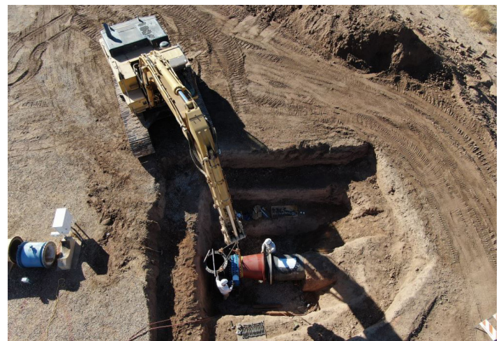
CAVSARP valve installation, Water Bank of Tucson
