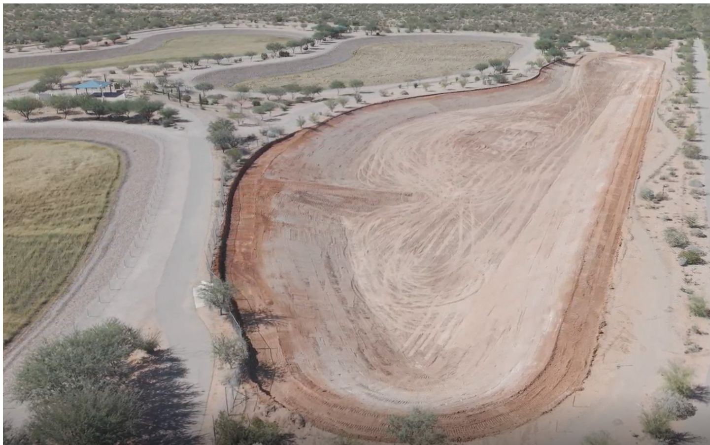
Construction of the 4th recharge basin at SHARP
