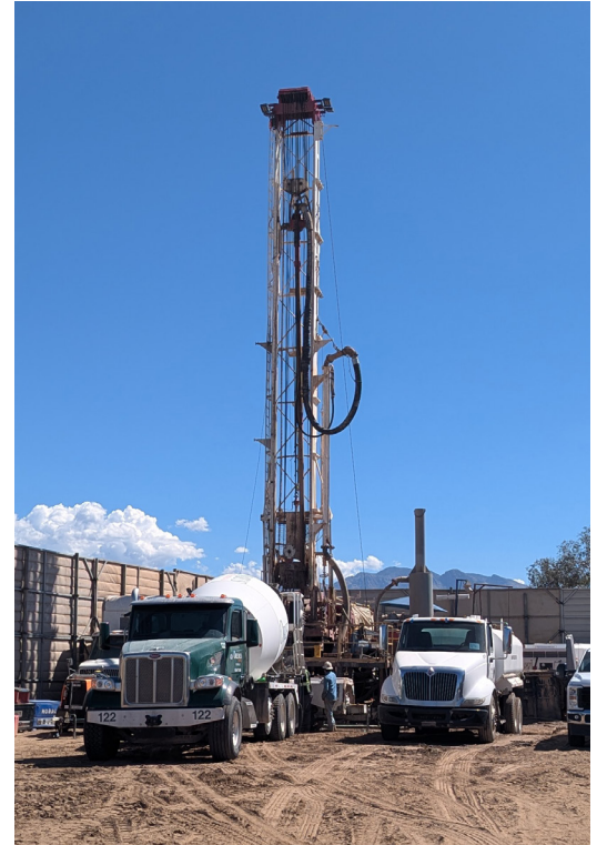
Drilling groundwater well Z-013B, Northwest Wells Treatment System Project
