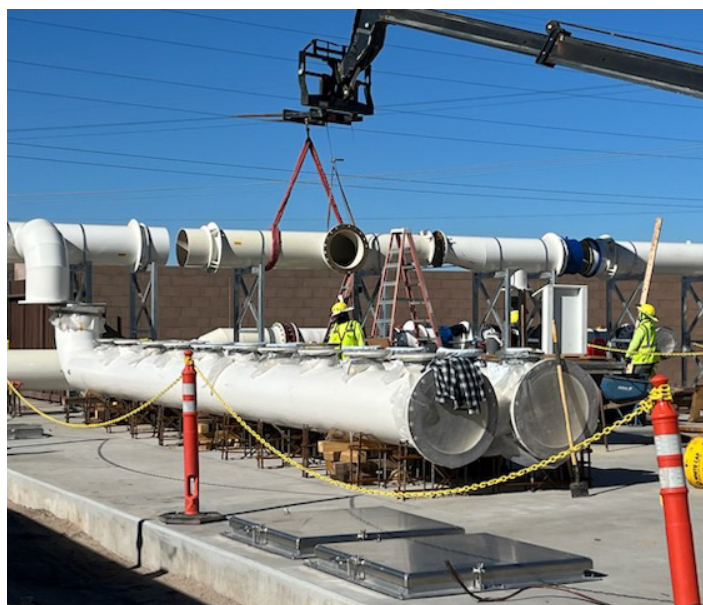
Installation of IX vessels at TARP
